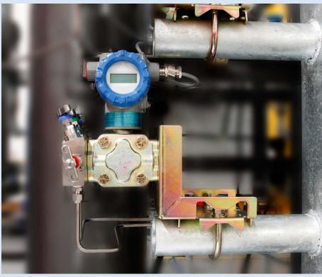
5) If your transmitter is to be installed outdoors or in a corrosive environment, make sure it appropriately sealed and protected.
