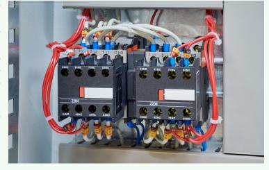
Contactor overheating, which results in severe pitting or deformation of the contact surface, can occur if too much current is transmitted, if the contactor does not close quickly and firmly, or if it opens too frequently. Once this happens, operation will become erratic and failure will be swift. Chattering, humming, and buzzing are common symptoms of contactor problems, and the stress of chattering can be a cause of failure in and of itself.
